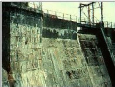
As the temperature drops below zero the water freezes causing the concrete surface to crack and break up.
